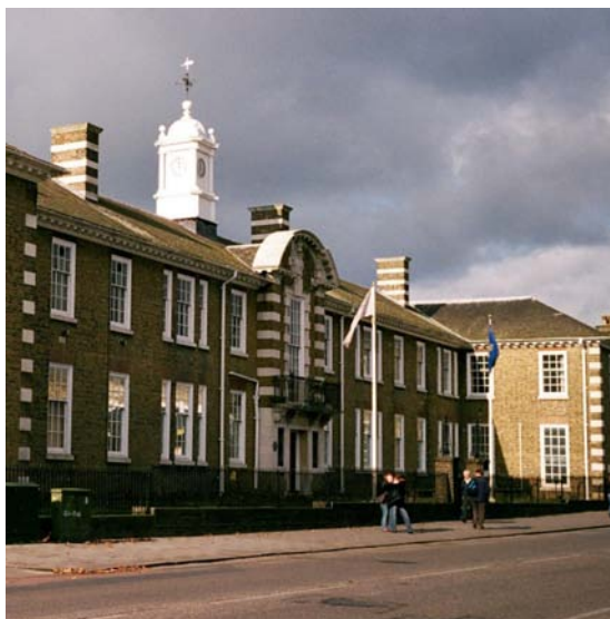
Above: Marconi's New Street Works dates from 1922. This was the world's first purpose-built radio factory and scene of the world's first radio broadcast by Dame Nellie Melba in 1920.
